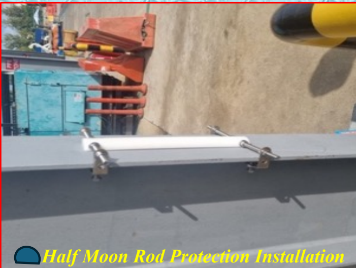
Corrosion Under Piping On Support Structure
