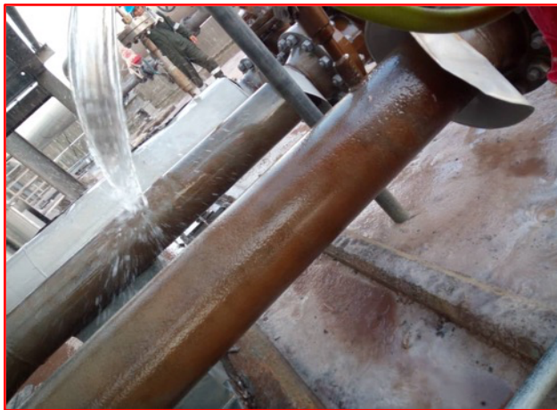
Wet Abrasive Blasting - HOT OIL CORROSION UNDER INSULATION
