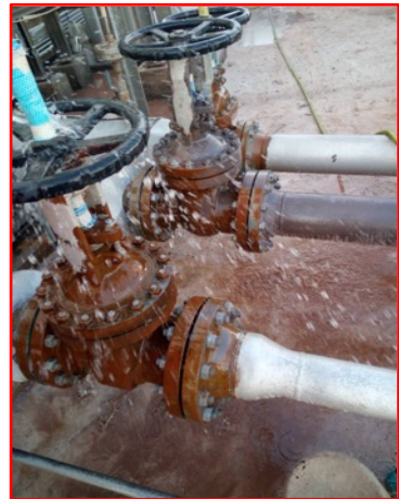
Wet Abrasive Blasting - HOT OIL CORROSION UNDER INSULATION
