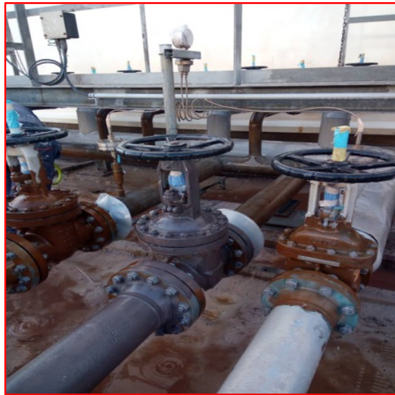
Painting - HOT OIL CORROSION UNDER INSULATION /HIGH TEMPERATURE PAINT
