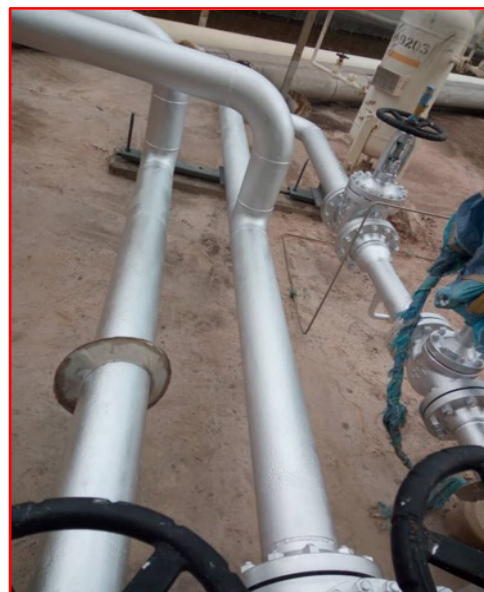
Painting - HOT OIL CORROSION UNDER INSULATION /HIGH TEMPERATURE PAINT
